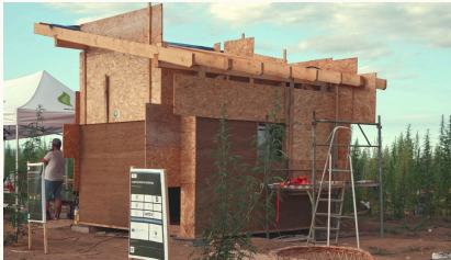
The demonstrator pavilion during construction, beside the hemp plots. Cast hemp–mineral walls, unfinished.
